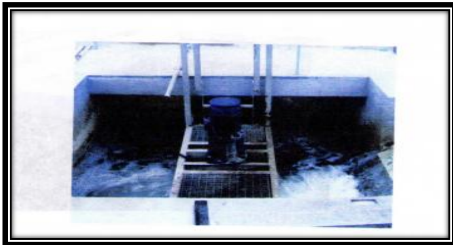
Figure (IV-4) : Bassin coagulation.
