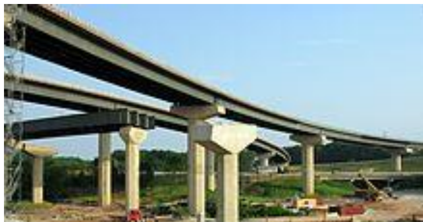
Figure1.3: Pont Baltimore (USA, 2008)
