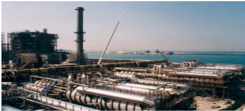
Figure III.4: Distillation (MED), Bahreïn [24].
