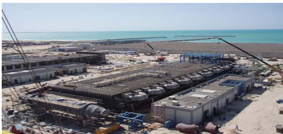
Figure III.6 : Distillation (MSF), Jebel Ali, Emirats Arabes Unis [24].
