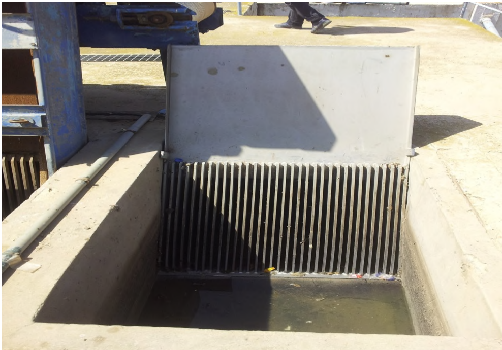
Figure II.6. Grille manuelle.
