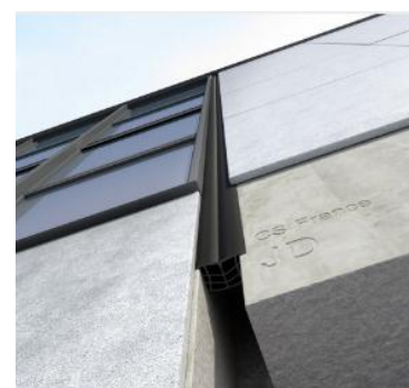
Figure 7: couvre joint des façades
