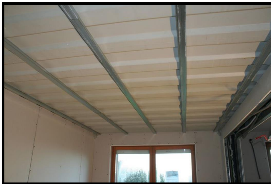
Figure 91: quadrillage de plafond
