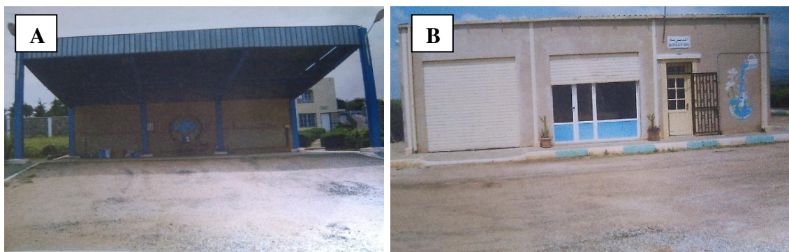
Figure 13: A: parking; B: Administration
