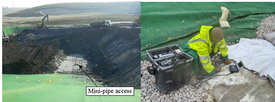
Figure4. View of the test pad and the insertion of the endoscope into the mini-pipe
