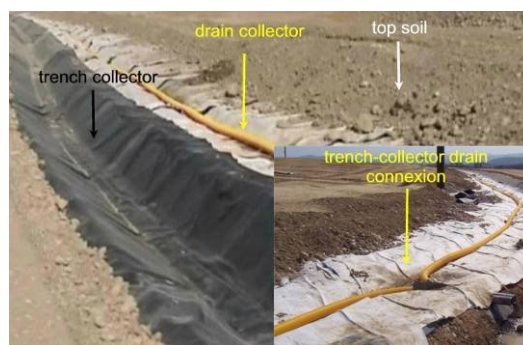
Figure13. Water collection system
