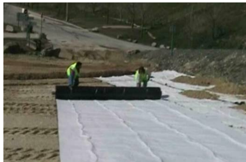
Figure12. Installation of the geocomposite on the top soil
