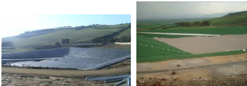
Figure9. View of the Landfill during work stage and after completion
