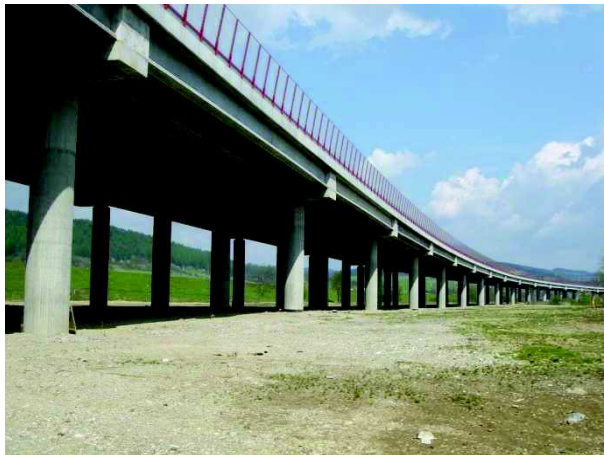
Figure 3. Concrete part of bridge structure
