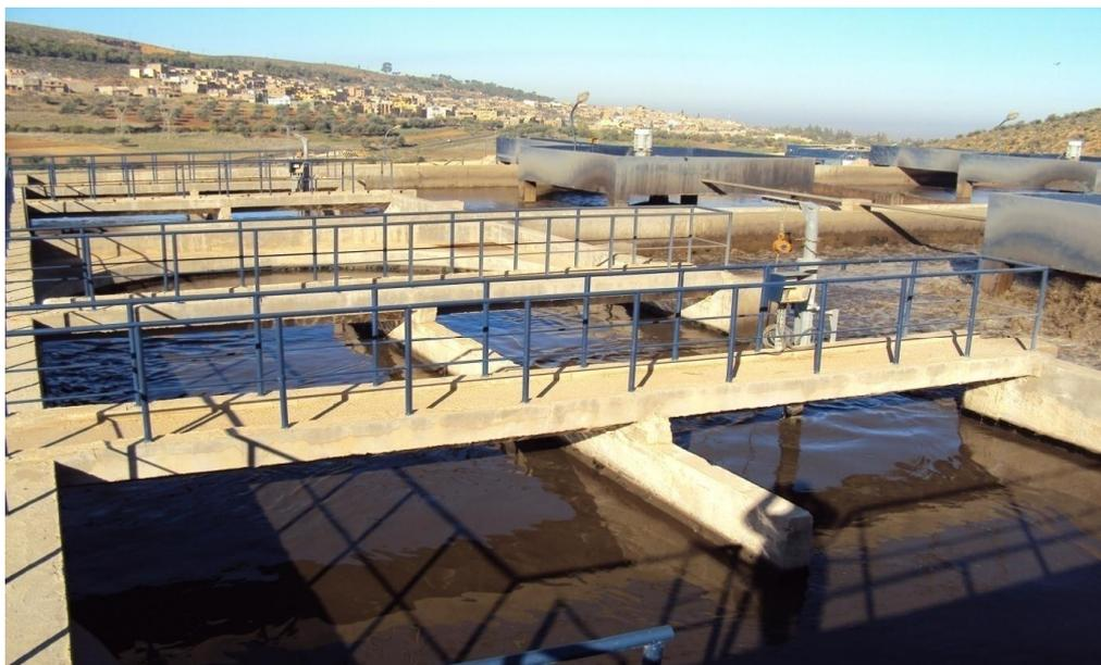
**Figure IV.8:** Bassin de nitrification dénitrification
