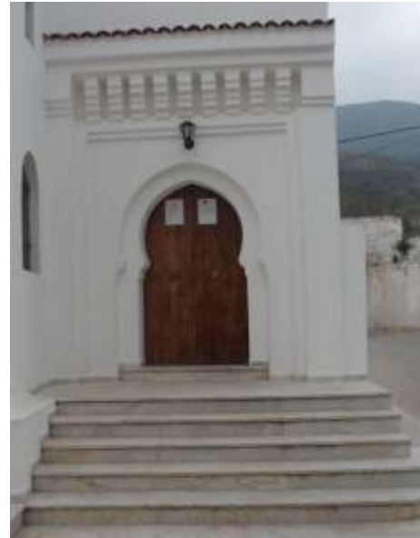
Figure 92: la porte ouest.
