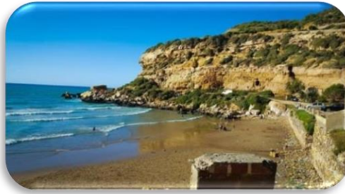
Figure 31: Station de Beni Saf.
