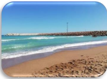
Figure 30: station de Beni Saf.
