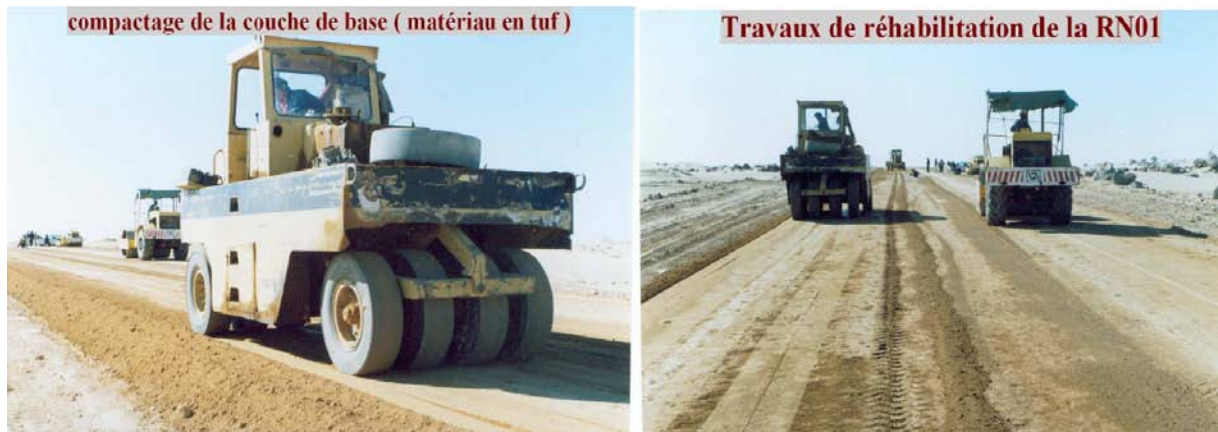
Figure I.4 – Renforcement de la RN01 entre Tamanrasset - In Guezzam (Sebaa, 2006).
