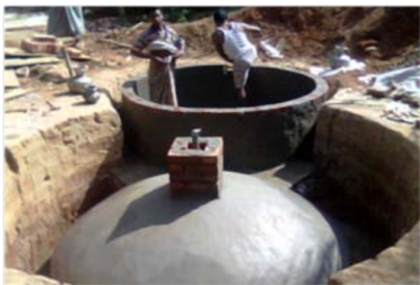
Fig. 5 : Construction of a biogas plant in a rural area of Bangladesh.
