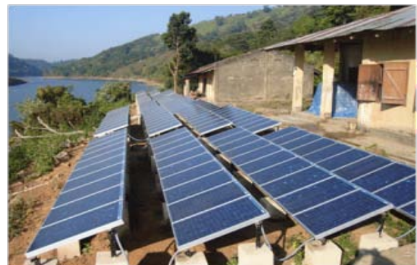
Fig. 3: Solar Arrays of 10 kW centralized AC market electrification systems at Barkal, Rangamati.
