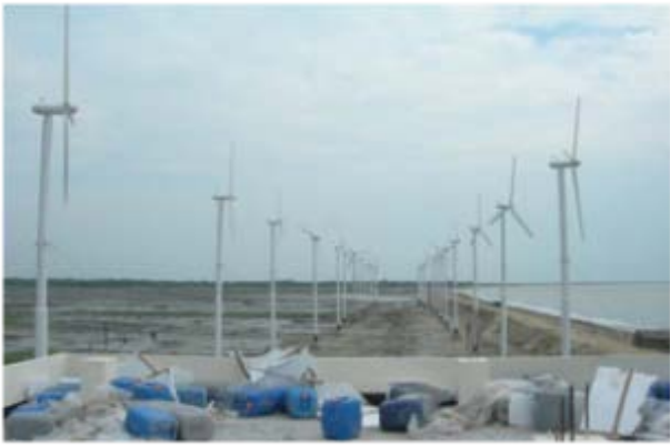
Fig. 4 : Wind turbines of 1000 kW capacity WBHPP at Kutubdia Island, Cox's Bazar district (Bay of Bengal).
