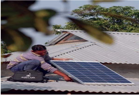
Fig. 1: Installing a solar PV system in a rural area.
