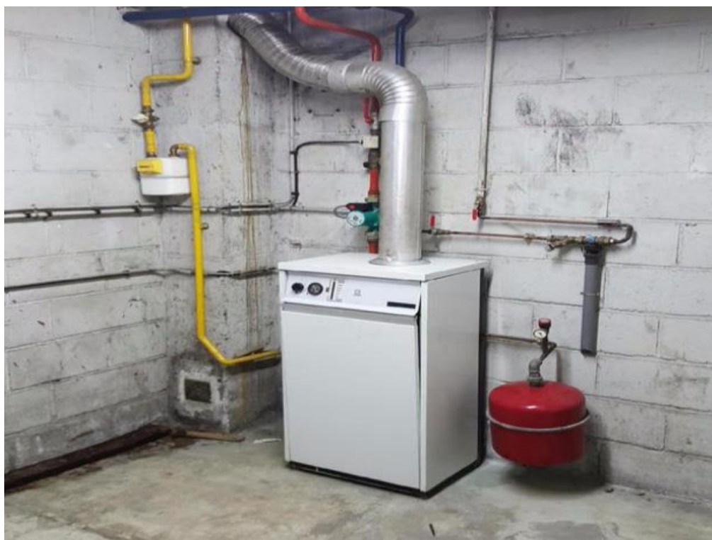
Figure 4. 2 - Chaudière au sol. [21]
