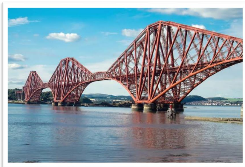
Figure 1- 24: Pont de Forth, Royaume-Uni
