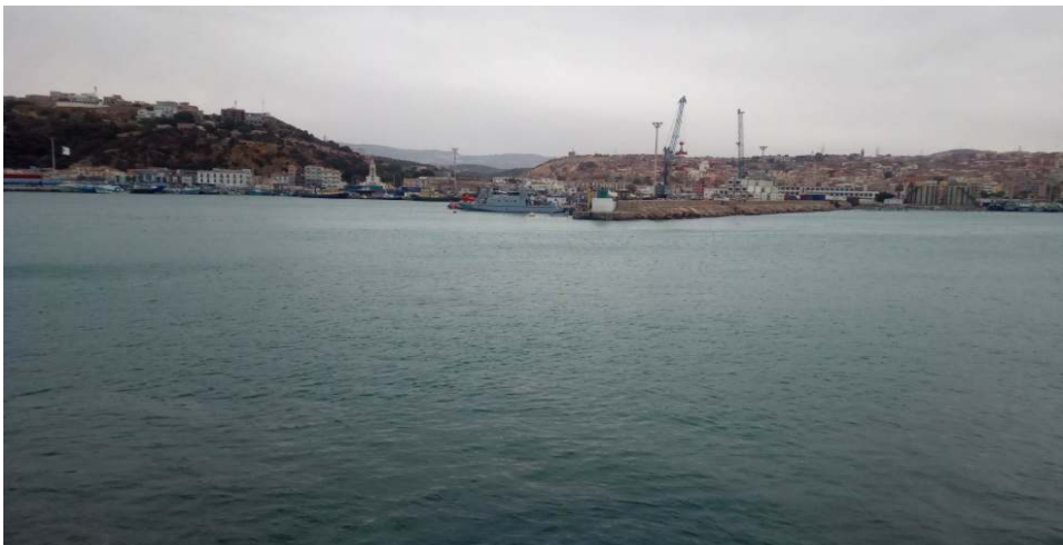
Figure 08: Le port de Ghazaouet (photo originale, 2023)
