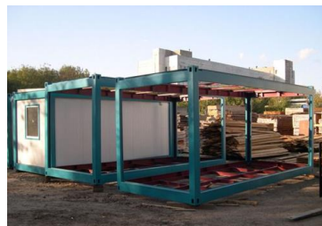
Figure 86: structure de container
