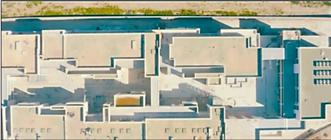
Figure 51 : Centre commercial GARDEN CITY.
