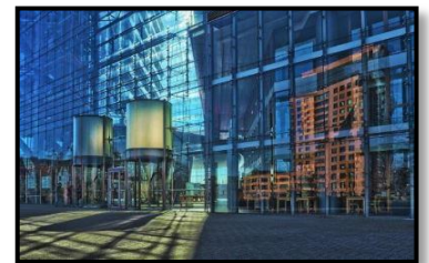
Figure 35 : façade non structurelle
