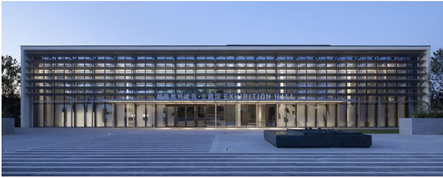
Figure 49 : façade sud de passive house pavillon
