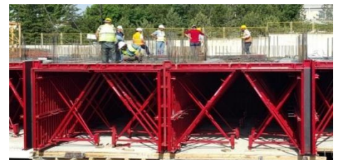
Figure 22: coffrage tunnel Source : (BAIRA 2019)
