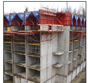
Figure 39 : coffrage tunnel (source : https://www.mesaimalat.com.tr/wp-content/uploads/2018/01/ERTF-1.jpg )
