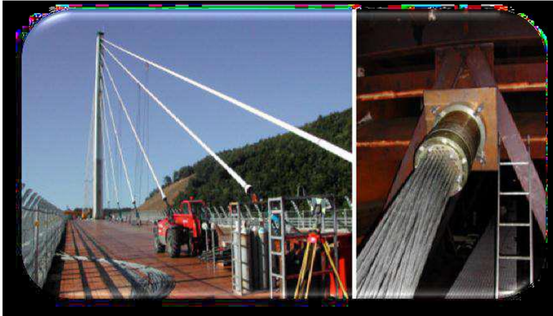
Figure I- 18: Configuration des haubans
