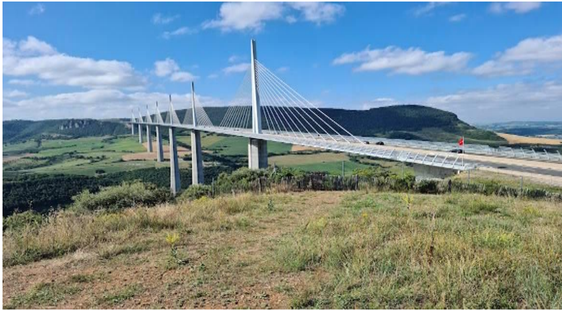
Figure I- 6:Viaduc de Millau France
