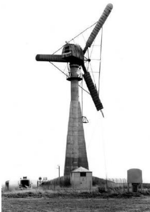
Figure 2.13 The Gedser Turbine.
