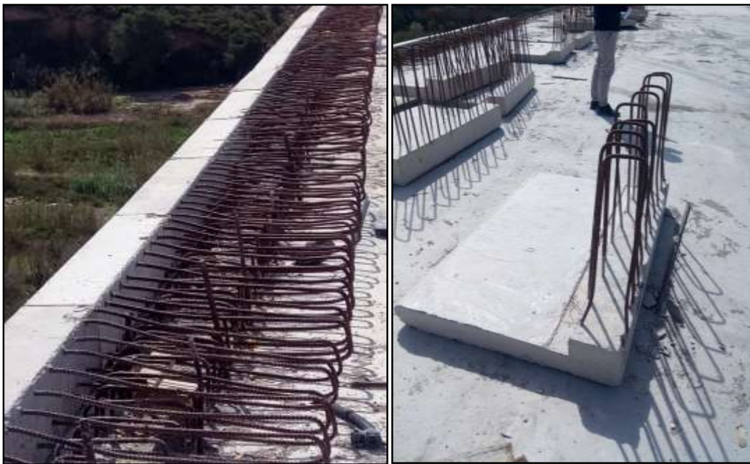
Figure 62: La pose des corniches
