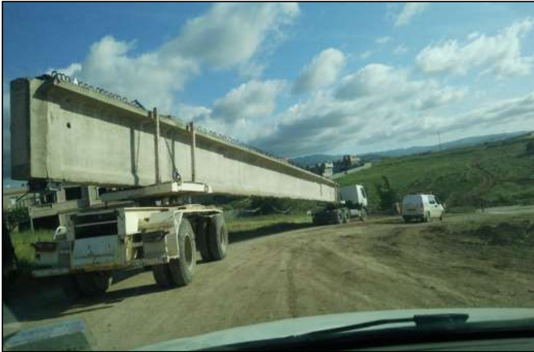
Figure 65: Transport des poutres
