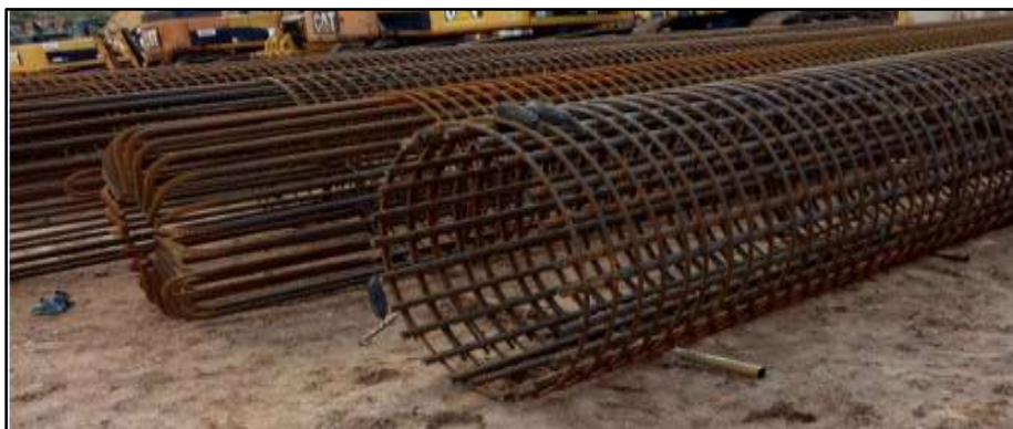
Figure 30: Cage d'armature
