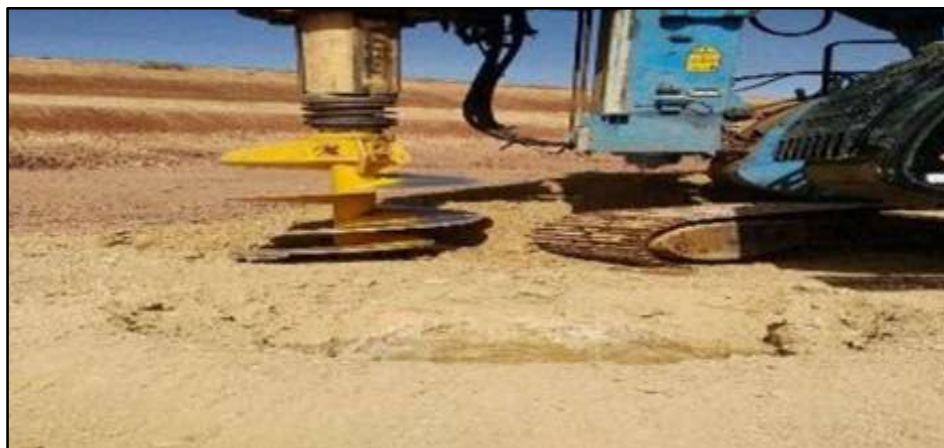
Figure 29: Forage du pieu
