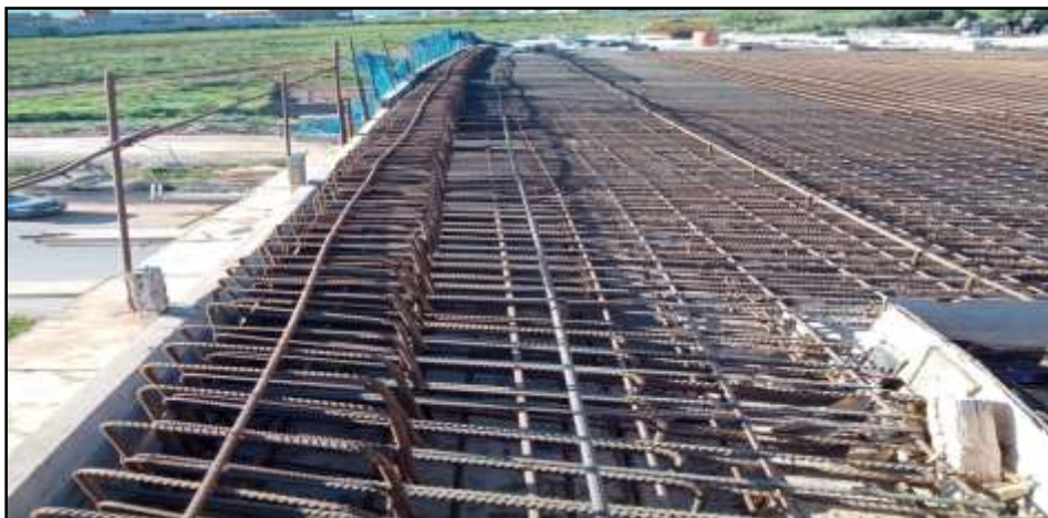
Figure 58: Ferrailage du portafons
