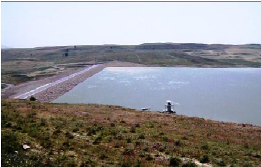
Figure 12: barrage d'Oued Athmania source (Mebarki,2008)
