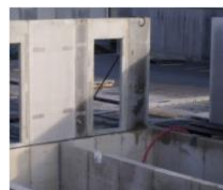
Figure 56 : Cloison béton isolant Source : http://www.sbp-prefa.com/panneau-beton/
