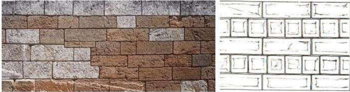
Figure 42. Description technique d'Opus quadratum
