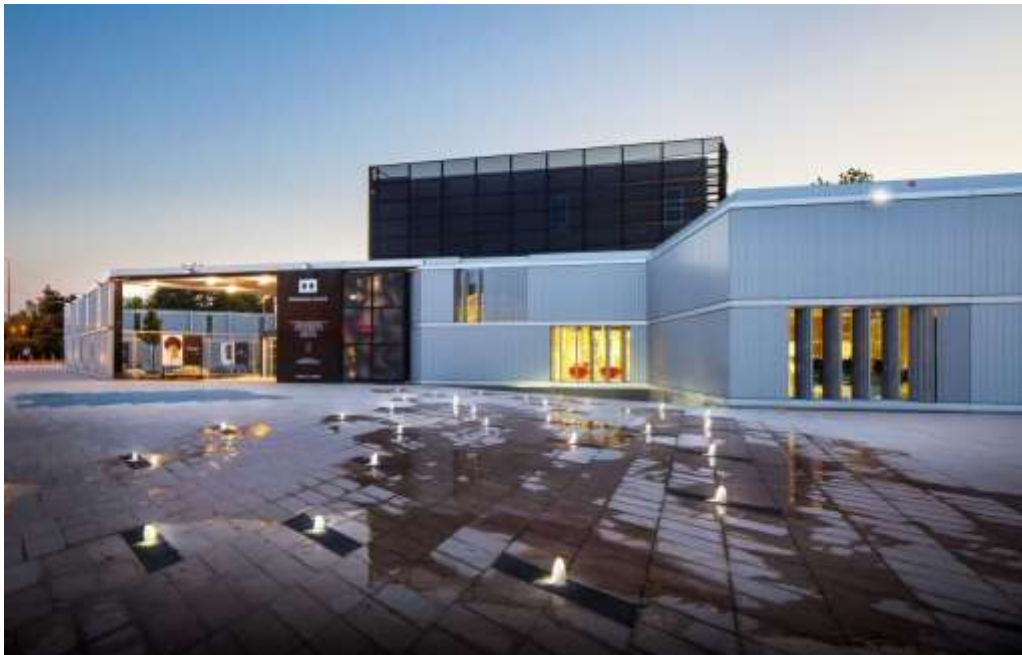
Figure 32: Médiathèque grand M / France
