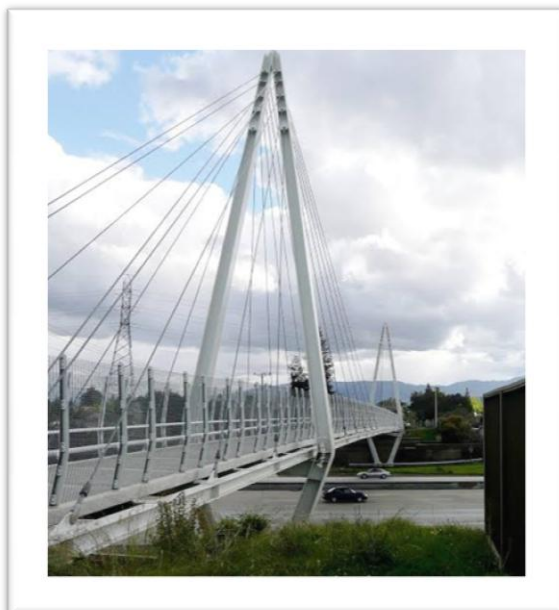
Figure 7 : passerelle a câble
