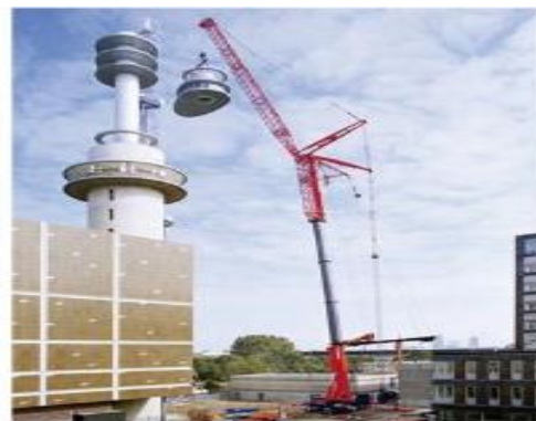
Figure 9 : Grue mobile LTM 11200-9.1 Liebherr
