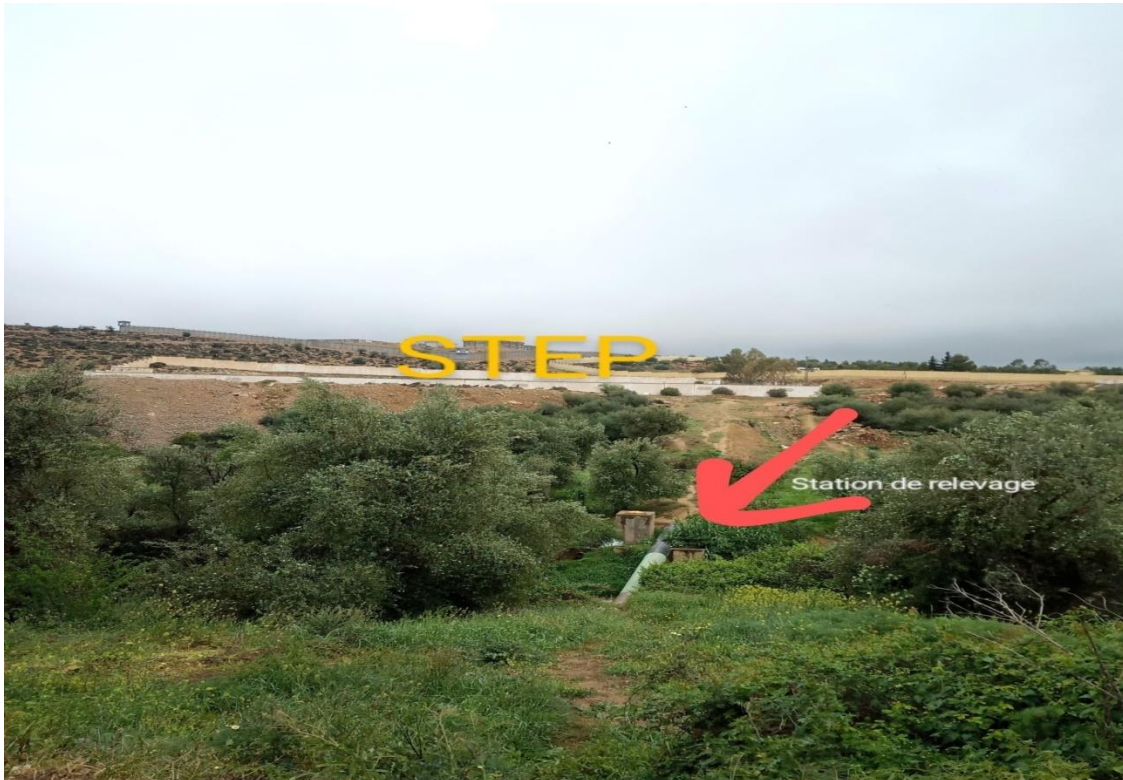
Figure IV.2. Photo position de station de relevage.
