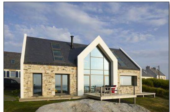
Figure8: Maison en pierre Source( https://www.google.com/search?q=choix+de+mat%C3%A9riaux+bioclimatique&rlz=1C1CHBD_frDZ888DZ888&hl=fr&sxsrf=ALeKk01SjiX6Lga-WD9x0rLqEk-KiCO6w:1616029310629&source=lnms&tbm=isch&sa=X&ved=2ahUKEwienIa00rjvAhUHnBQKHRHzAaIQ_AUoAXoECAEQAw&biw=1920&bih=969#imggr=sghZXfwyx47R6M&imgdii=MX0xxStI68JdM )
