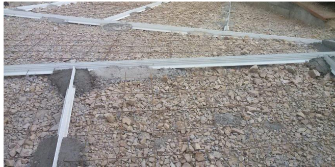
Figure 124. Joint de dilatation 181
