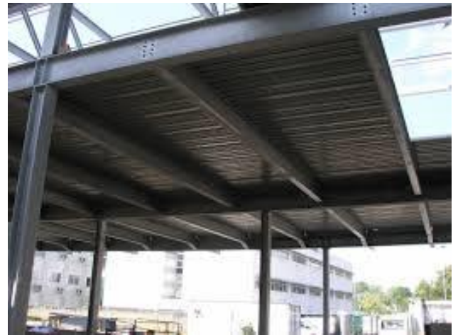
Figure 119: plancher collaborant / source : google image.
