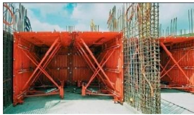
Figure 37. Le coffrage tunnel
