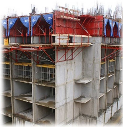
Figure 1 : coffrage tunnel 1
