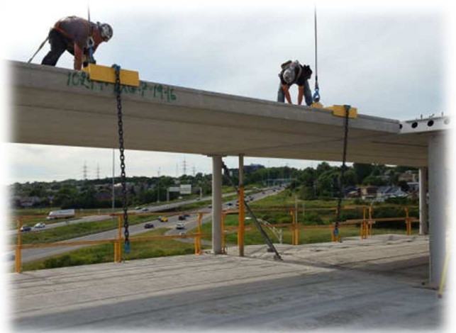
Figure 65: assemblage dalle poutre
