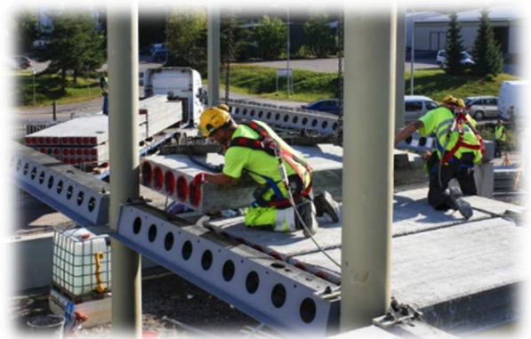
Figure 57: l'installation du DELTA BEAM
