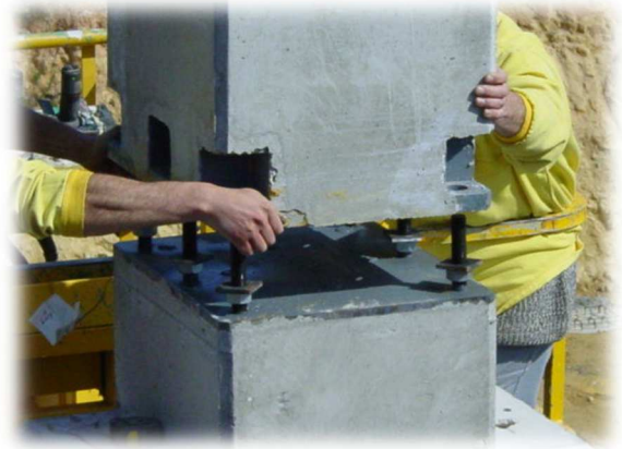
Figure 47: la connexion poteau-poteau
