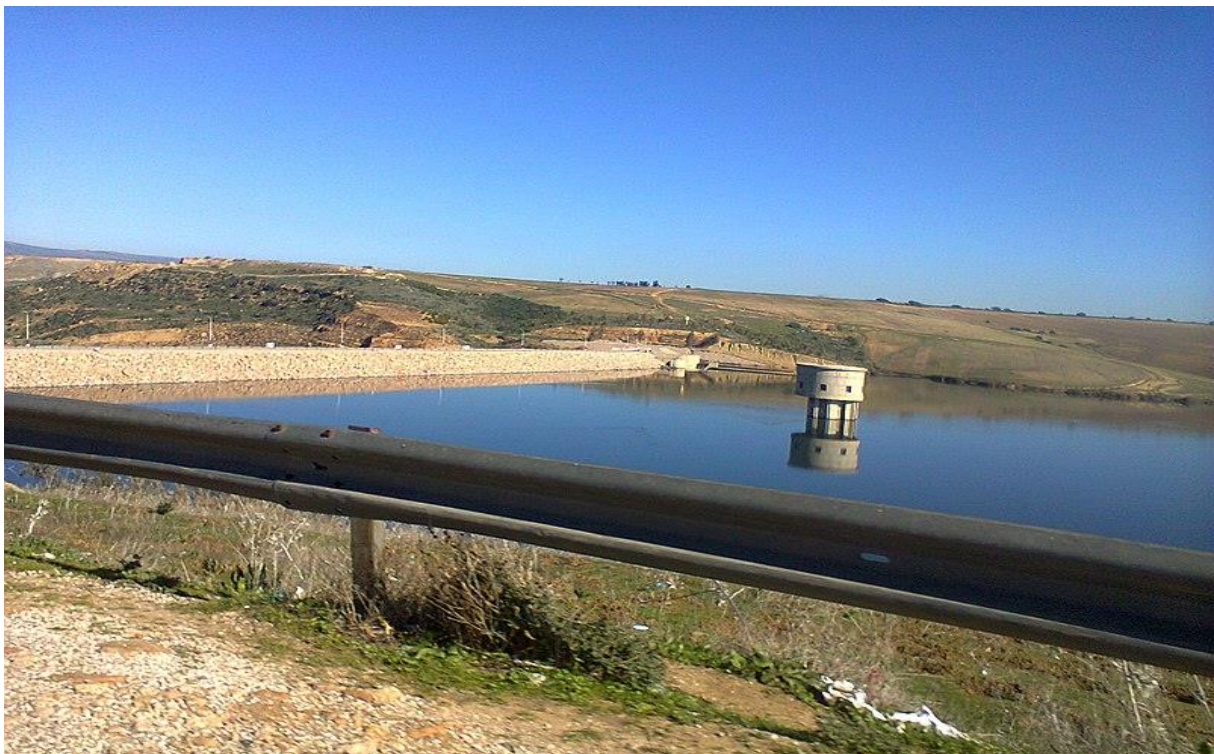
Figure III.11 : photo Barrage de Sikkak [6]
