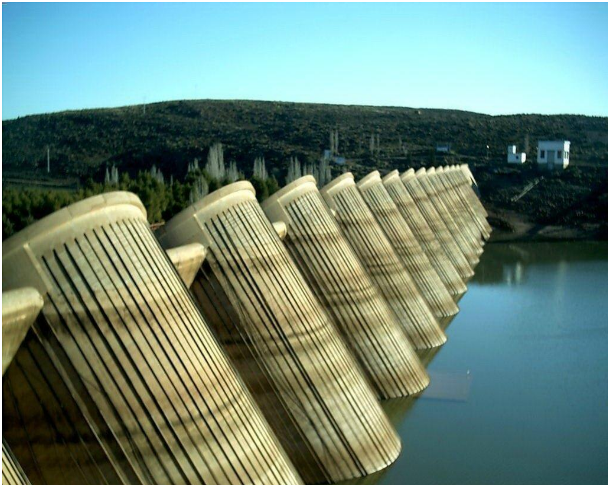
Figure III.18 : photo barrage de Meffrouche [17]
