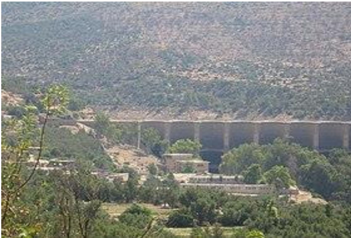
Figure III. 8 : photo barrage de béni Bahdel [5]
