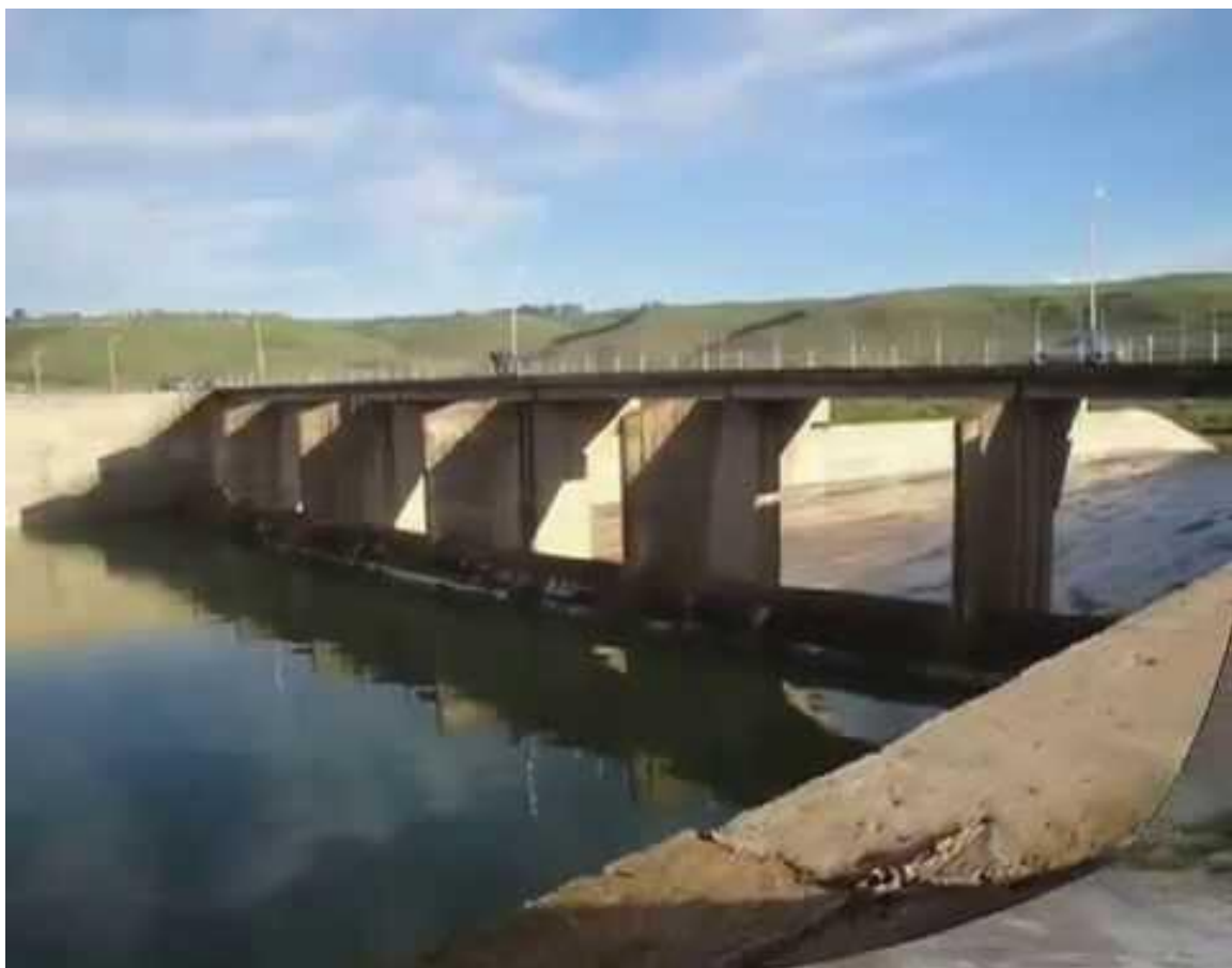
Figure III.15 : photo barrage de Sidi Abdelli [15]
