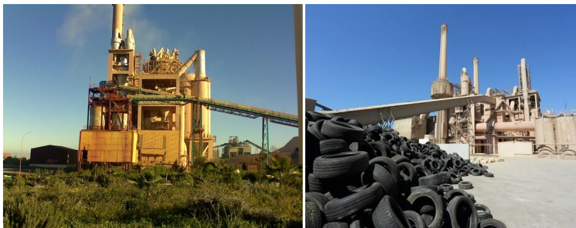
Figure 21: Bandes transporteuses (tapis roulant) Figure 22: Pneus usagés
