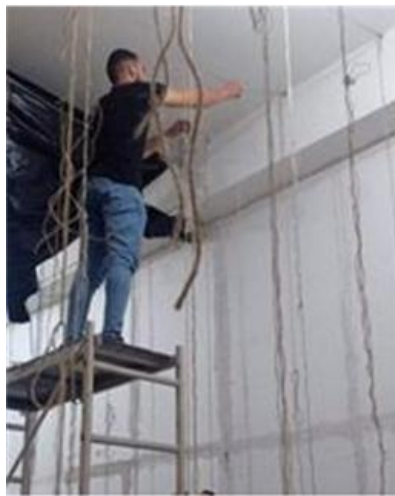
FIGURE 8: SUSPENSION DES CORDES (PHOTO ORIGINAL)
