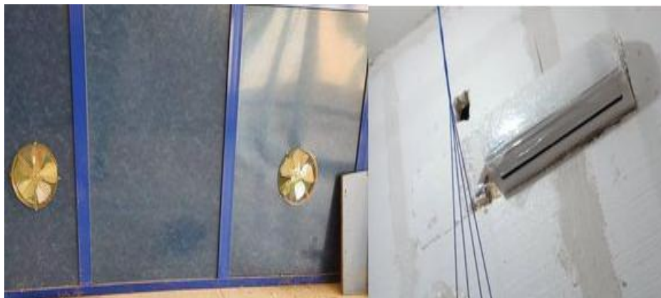
FIGURE 11: EMPLACEMENT DE VENTILATION ETCLIMATISATION (PHOTO ORIGINAL)
