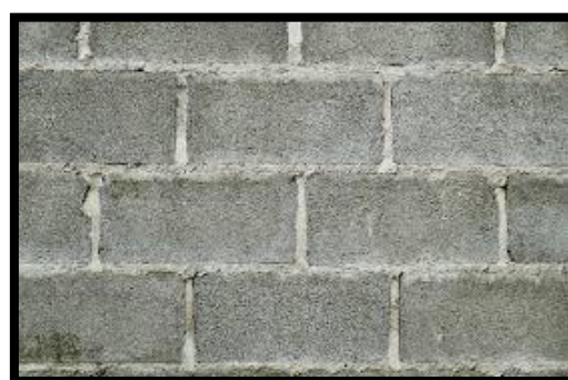
Figure 77 cloison en parpaing
