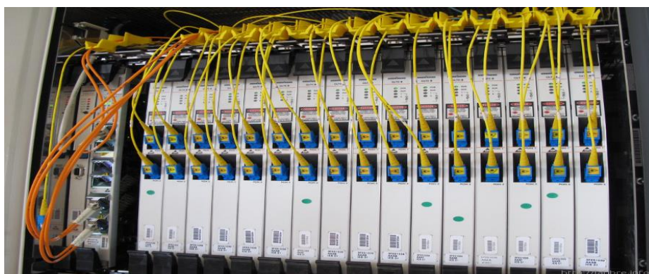
Figure II.5: Ligne optique terminal OLT
