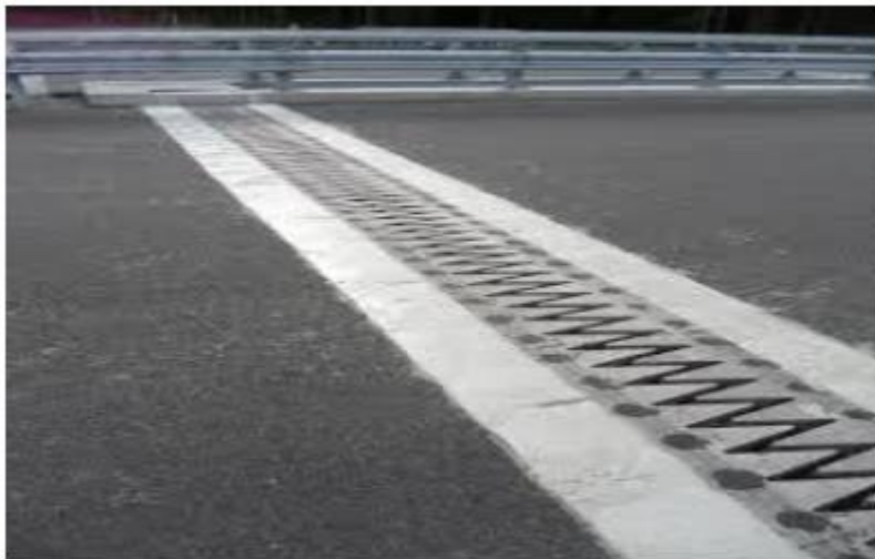
Figure 27:les joints de pose
