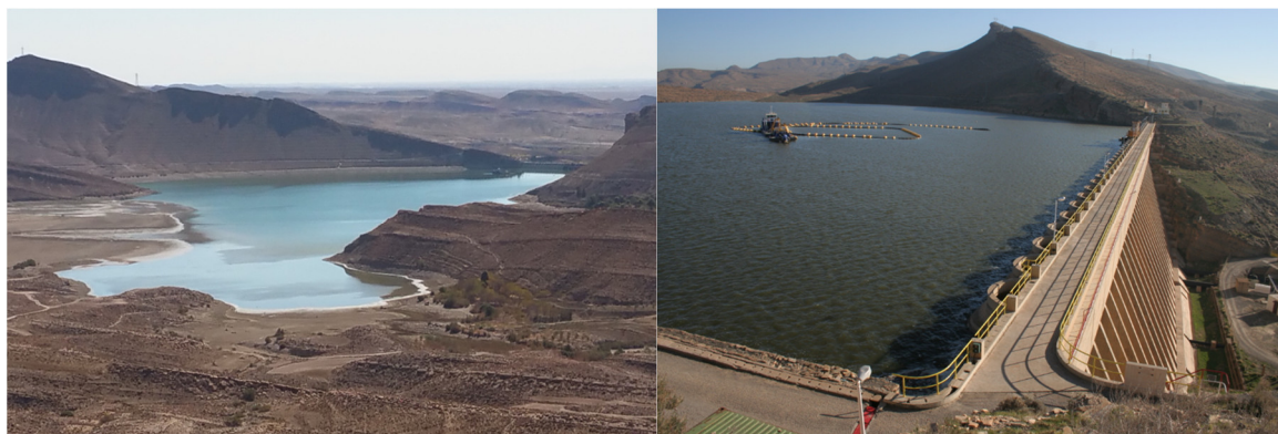
Figure II.17 Barrage K'sob (photo : Guesri 2016)
