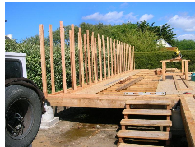
Figure 537 : Ossature bois Source : http://pailienfinistere.canalblog.com/archives/2009/05/18/13777809.html
