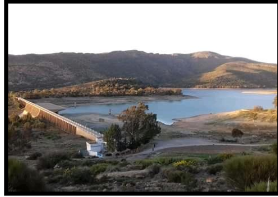
figure 06: Barrage de Beni Behdel
