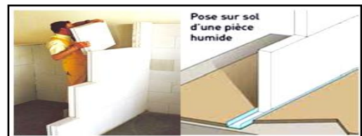
Figure77: La cloison SIPOREX
