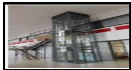
Figure 184: Monte de charge hydraulique
