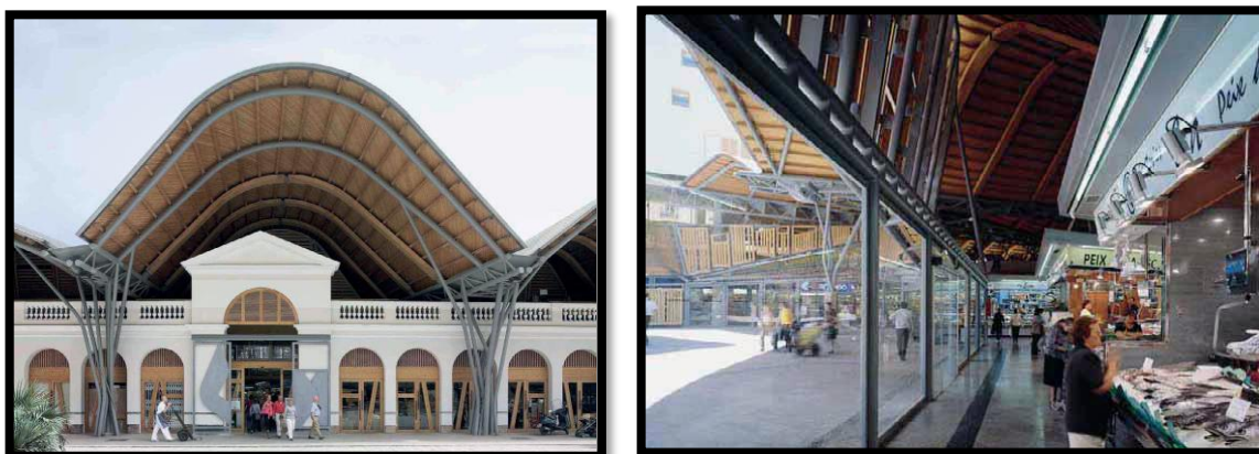
Figure 77. Galerie commerciale Santa Caterina Market, Barcelone
