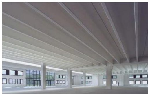
Figure 101: plancher nervuré
